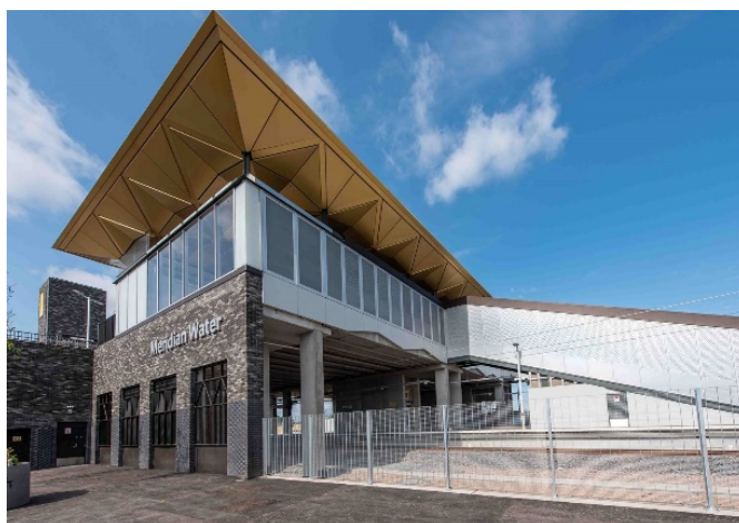
Meridian Water station, completed (2019)
